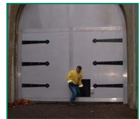
Workers must first enter through the small access door to get to the latches.
