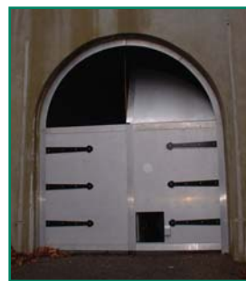
Workers must first enter through the small access door to get to the latches.
